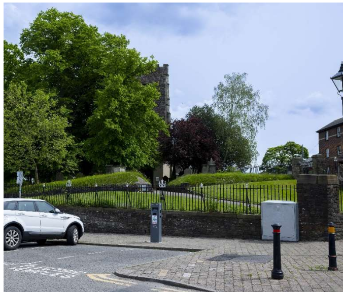
On Street Charging at St Woolas
