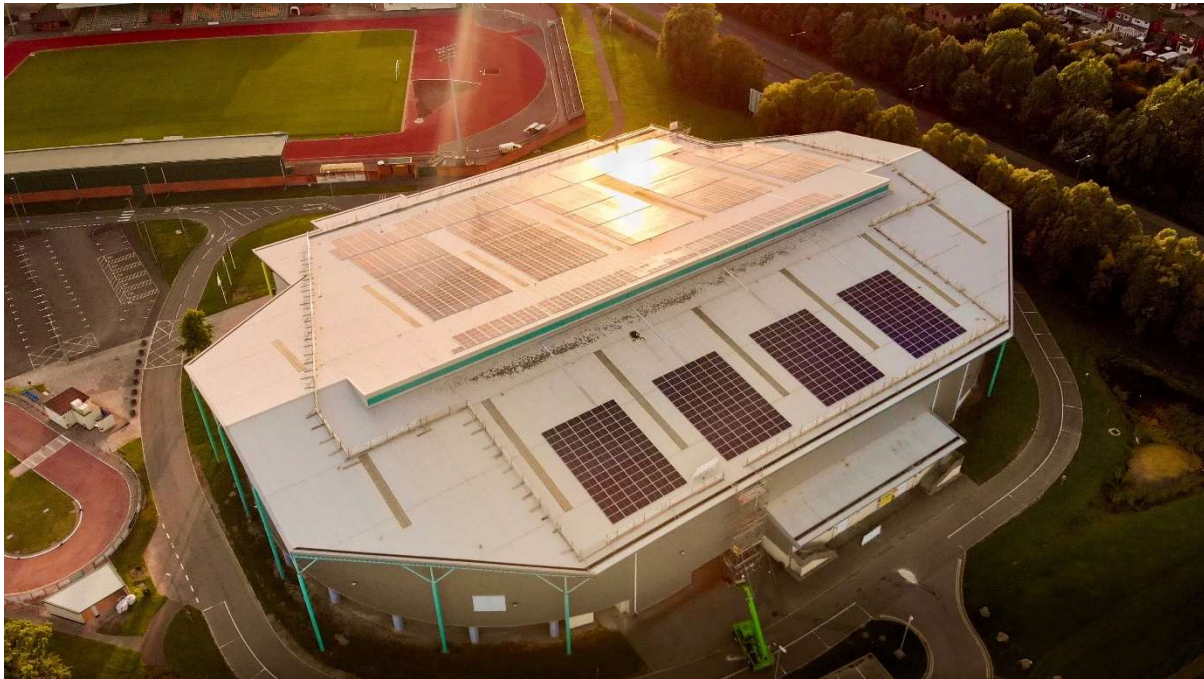
Solar panels on the roof of the Newport Geraint Thomas Velodrome
